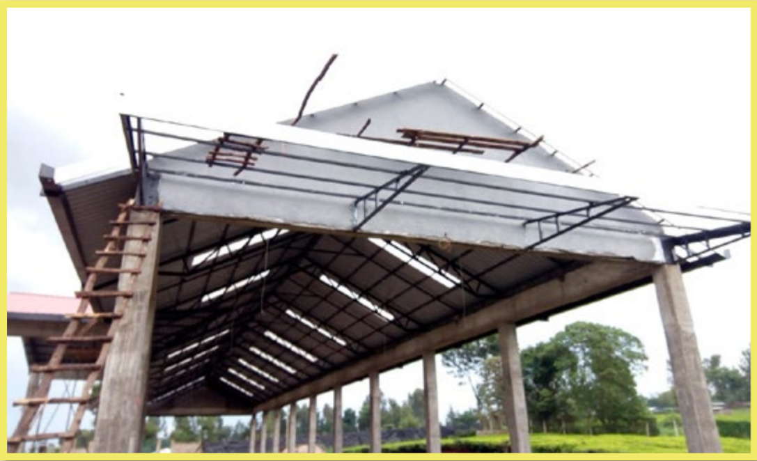
Roofing in progress DD/MM/YYY
