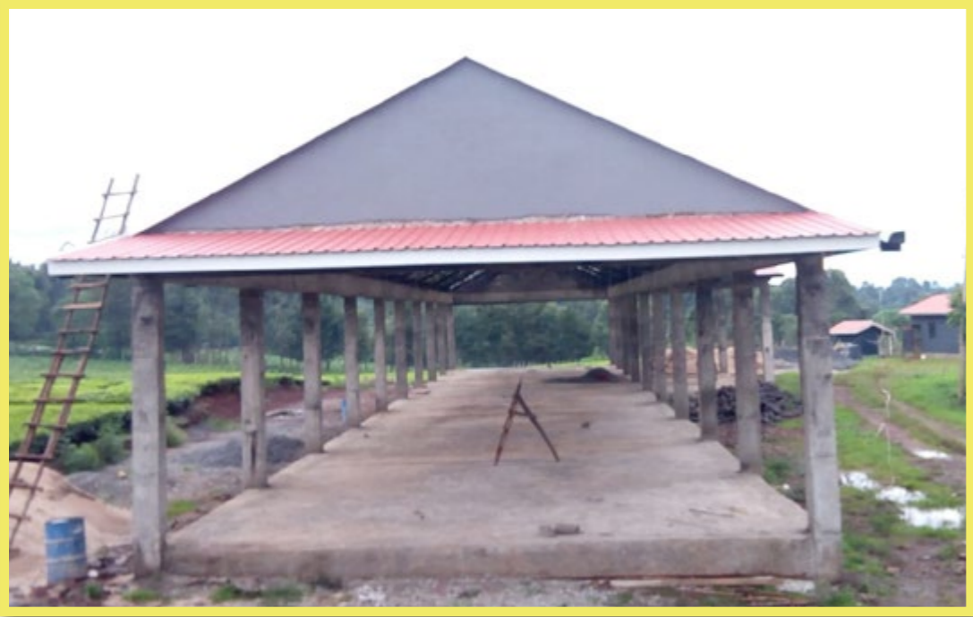
Roofing is complete DD/MM/YYY
